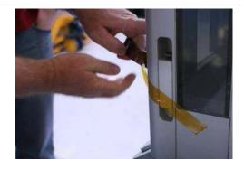
Prepare the box and foam. Note the cutout in the foam which aligns with the rear of the enclosure.
